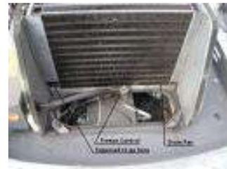
Soak the coils well- if there is a lot of crud on them, use a bristle brush to clean the coils- carefully, as the fins are delicate, to scrape off the crud. Another option is using a "fin comb", which is also good if the fins are bent, restricting the air flow.
