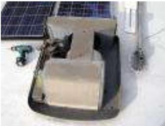
The evaporator cover (if it's metal) will be attached by a number of sheet metal screws, remove these, but **pay attention to the screws as you remove them**. On some models there will be either different length screws, some screws might be blunt ended to go in to electrical areas. Just pay attention and replace the screws in the same way they were removed.
