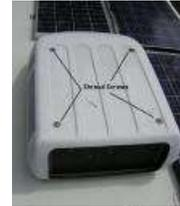
Once you have the shroud off, you have to get to the evaporator, which is the front of the unit under a (usually) sheet metal (sometimes styrofoam) cover.
